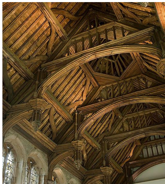
The roof of the Great Hall
